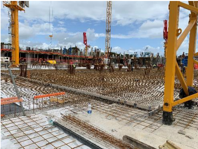
Cast insitu suspended floor
